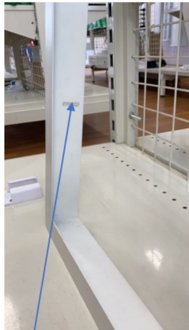
2cm x 0.5cm Distance between each hole site: 15cm : 45cm : 45cm : 15cm
